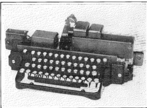
Creed Teleprinter with Keyboard Conforming Strictly to the Commercial Typewriter Layout.
